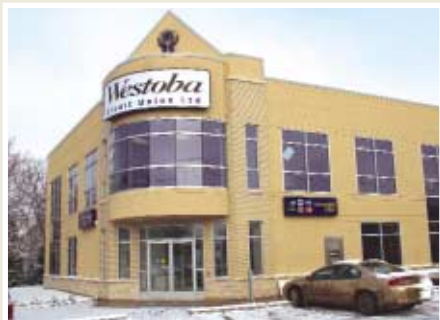
Newly renovated exterior
