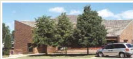
Killarney Branch, before renovations
